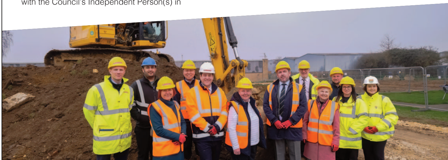
Council homes start to take shape, Wellington Way, Market Deeping
